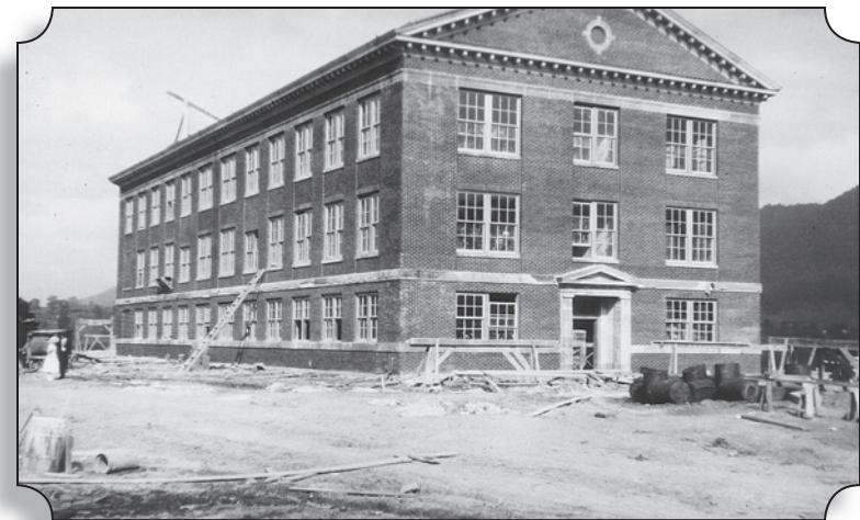
THE CONSTRUCTION OF LANSDPELL HALL, 1922, BC'S FIRST BUILDING.
