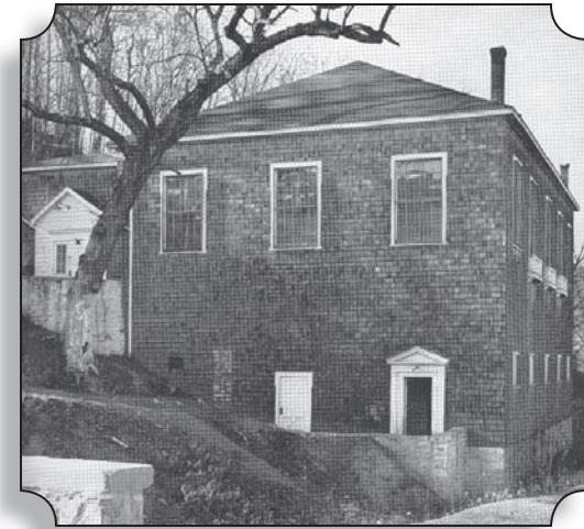
THE OLD GYMNASIUM, LONG SERVICED, 1947
