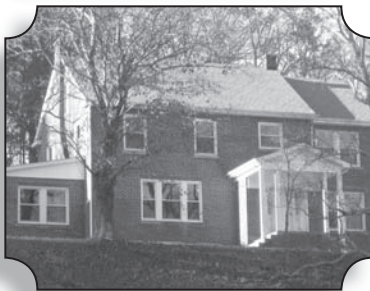
CONSTRUCTION (above) AND COMPLETION (below) OF BC’s NEW MISSIONARY-IN-RESIDENCE HOUSE.
